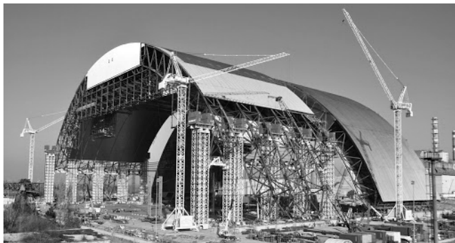
Fig. 28. Installation of confinement structures
